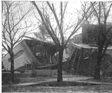
A WIND STORM LOSS
